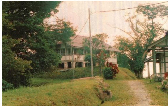
This building, the former Crag Hotel, was turned into Uplands Primary School in 1955 and has lately been used as The Royal Simla Club in the Channel 4 series Indian Summers CREDIT: UPLANDS 40TH ANNIVERSARY MAGAZINE
